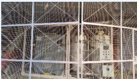
2 PSA plants of 750 and 1160 LPM capacity
